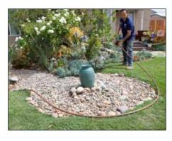
Using the same reliable self-dispensing coil as other XF Series Dripline tubing, the QF Header lays straight when uncoiled and is easy to install around non-linear landscape features. It bends to a 38 cm radius without damage or kinking.
